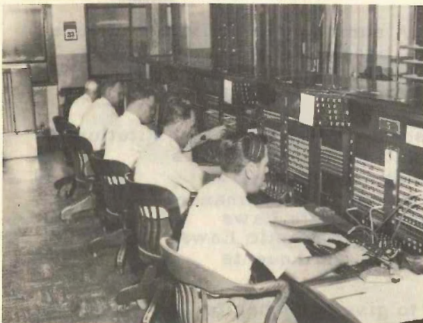
Central Headquarters Switchboard
